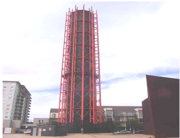
St. Melbourne 12-storey Vent stack
