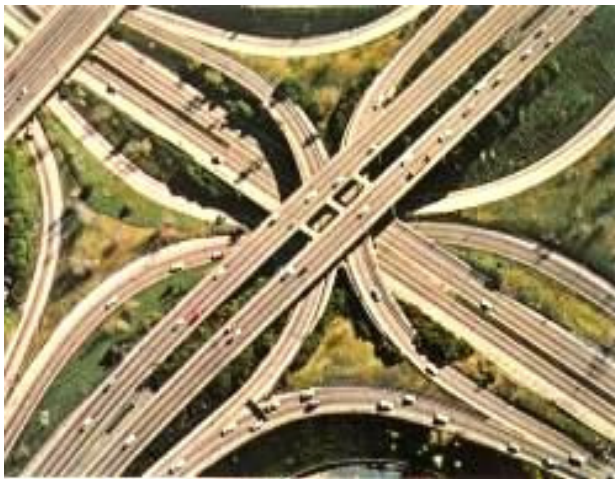
Los Angeles Spaghetti Junction
